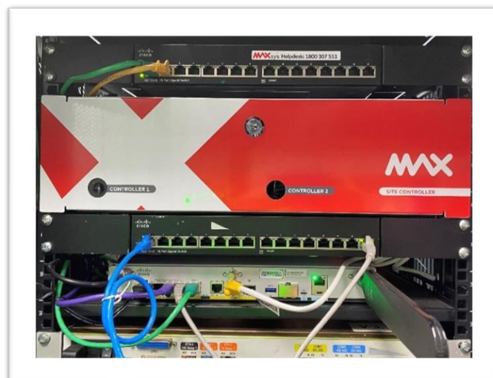
Fig 3. CMS Site Controller Rack
